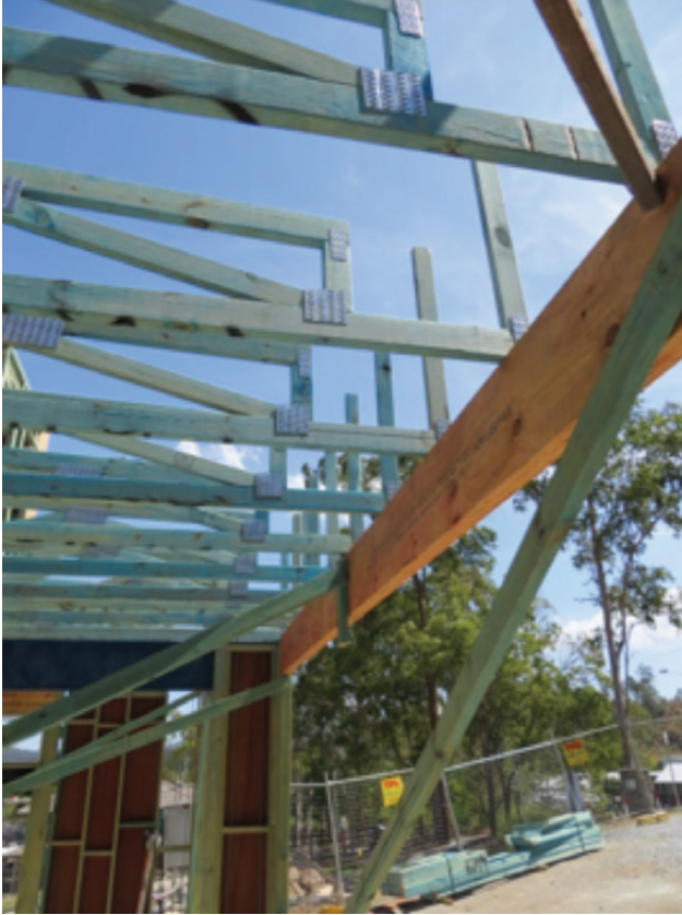
Photograph 11 – Structurally deficient parapets
